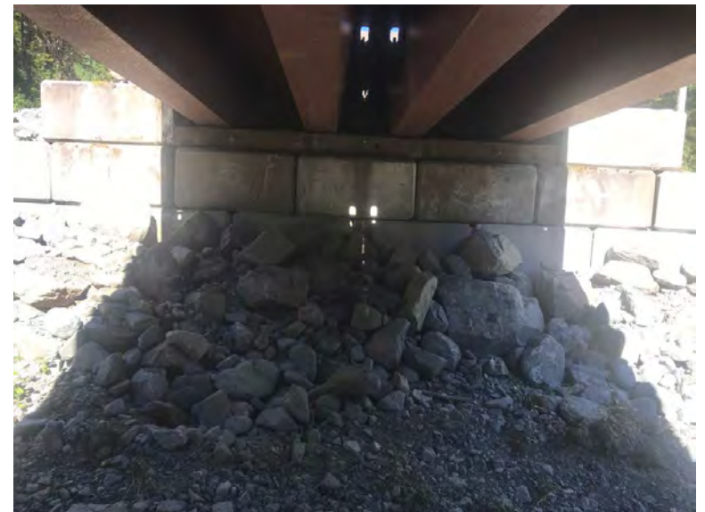
Left Bank Abutment when facing downstream
