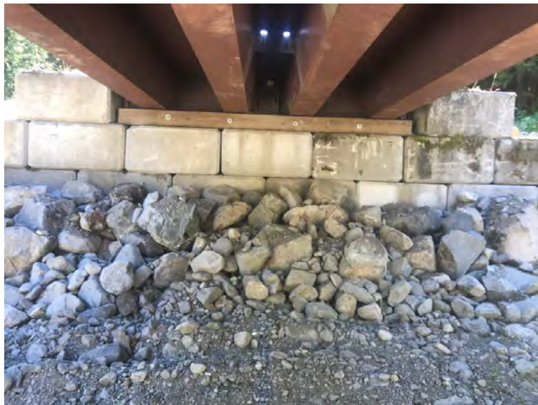
Left Bank Abutment when facing downstream
